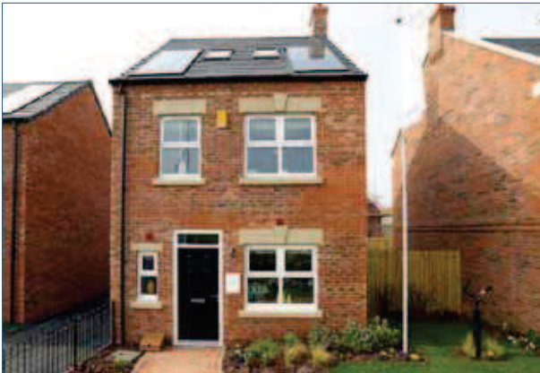
Farndale Housing Development
